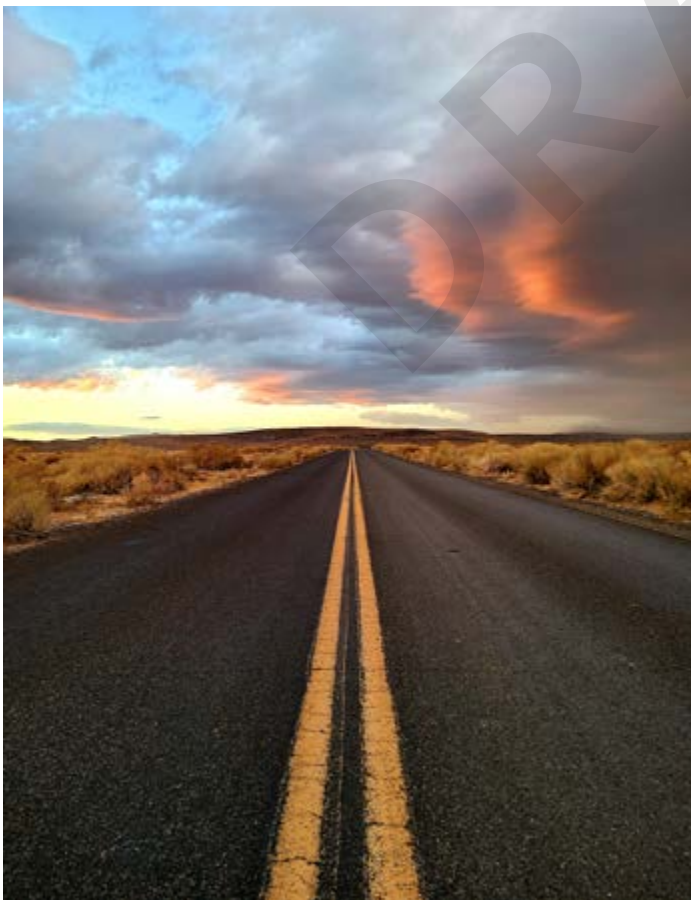
Paved main road
