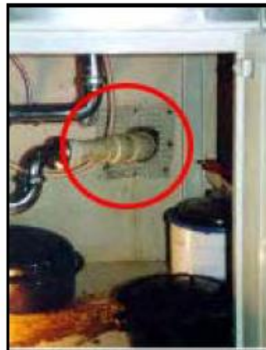
Use lath metal around pipes
