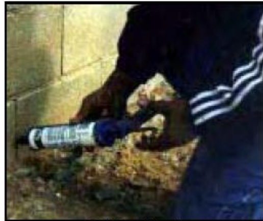
Seal holes with caulk
