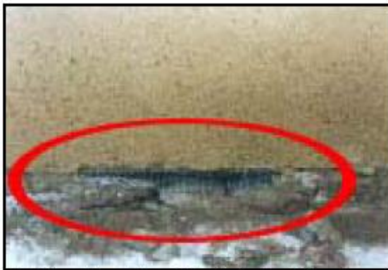
Fold lath metal and place in holes in the foundation of houses
