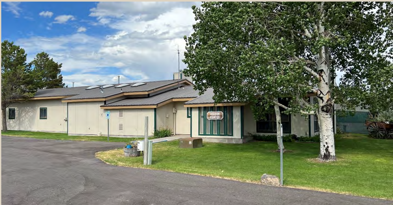
Exterior view of the visitor center/ranger station.
