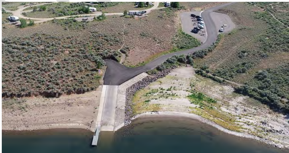
View of the current boat launch facility and parking area.
