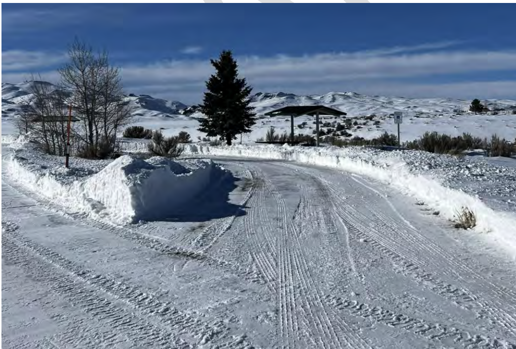
Paving site pull-outs and the loop road in Campground Loop #2 will allow WHSRA staff to more efficiently remove snow in the winter, helping ensure the facility is open year-round.
