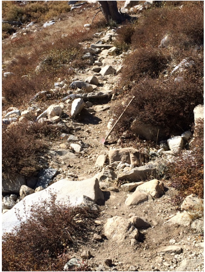
Examples of trails impacted by erosion that will need drainages constructed, as well as tread surface improved for user safety.
