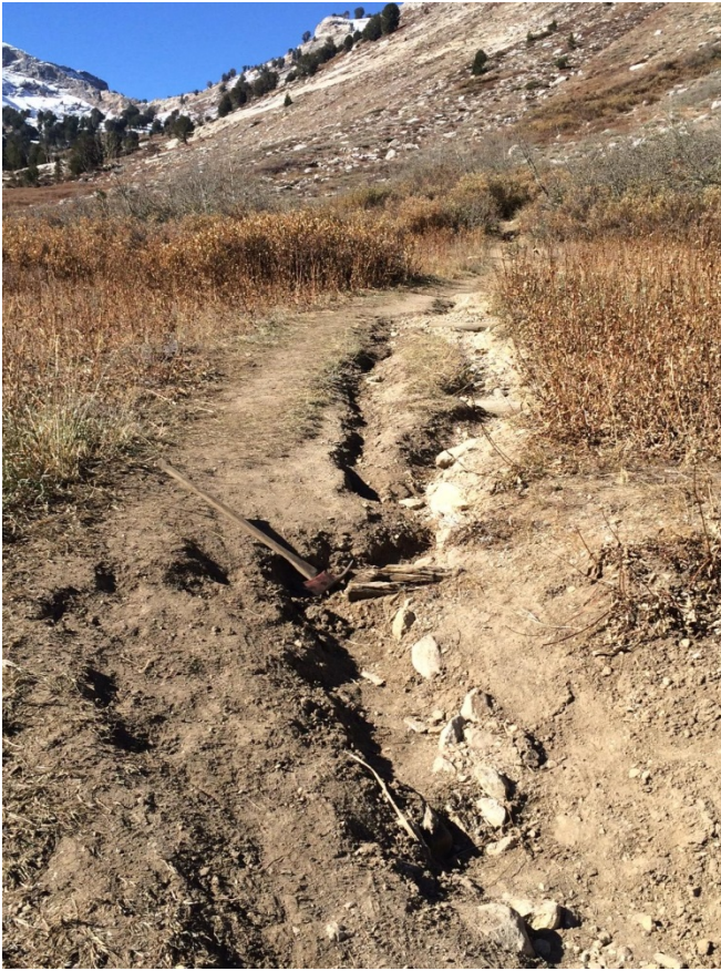
Examples of trails impacted by erosion that will need drainages constructed, as well as tread surface improved for user safety.
