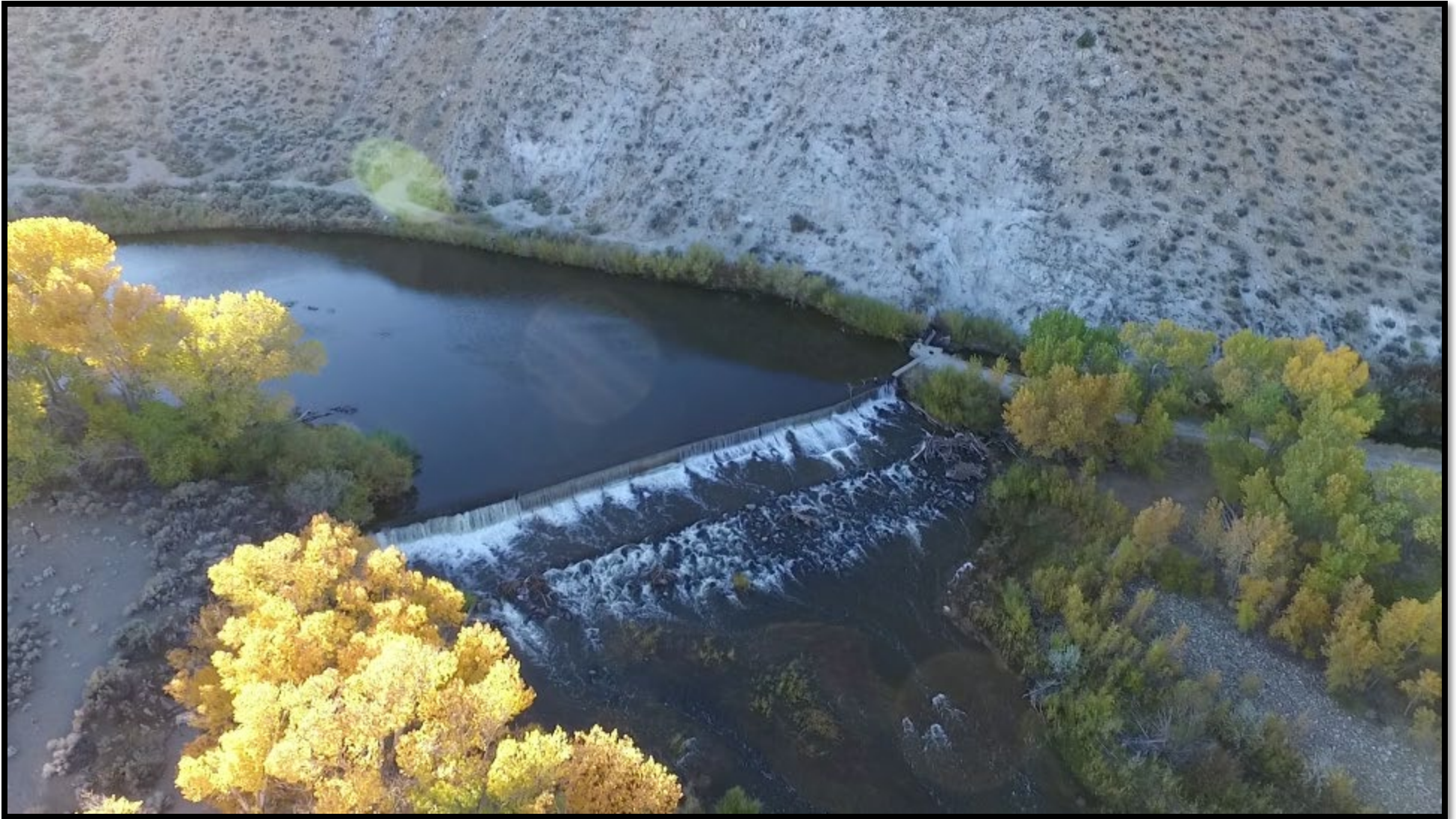
1 Site of Mexican Dam Portage
