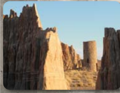
C.C.C. Water Tower
